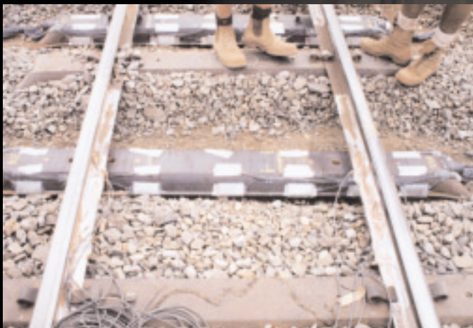
Installation of Instrumented Sleepers at QR
