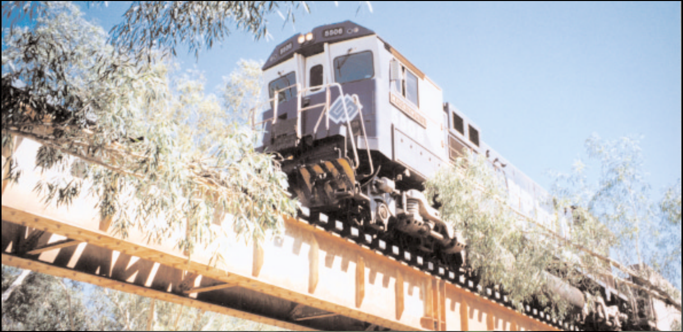
Steel girder Bridge on BHP-IO Goldsworthy Line
