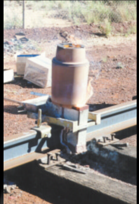
Aluminothermic welding
